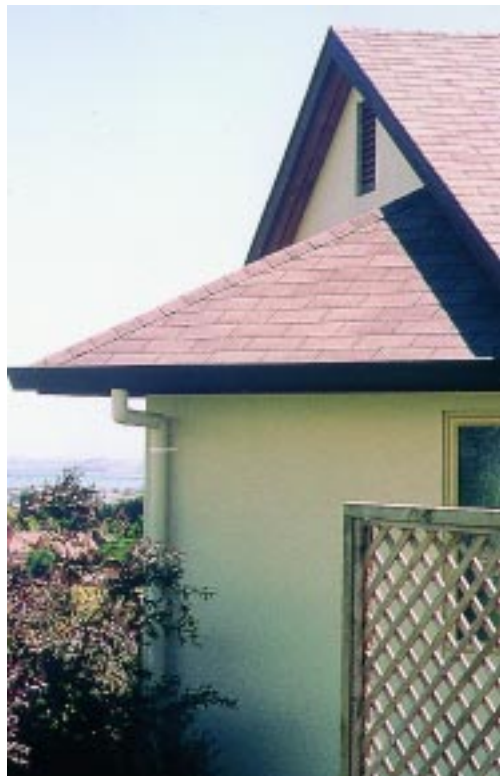
Centre vent in gable
