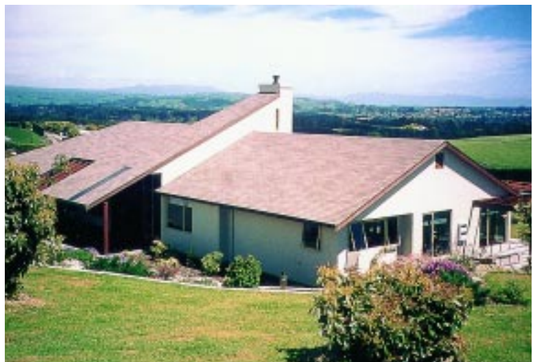
Vent near chimney
