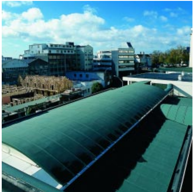
Rubber membrane on plywood
