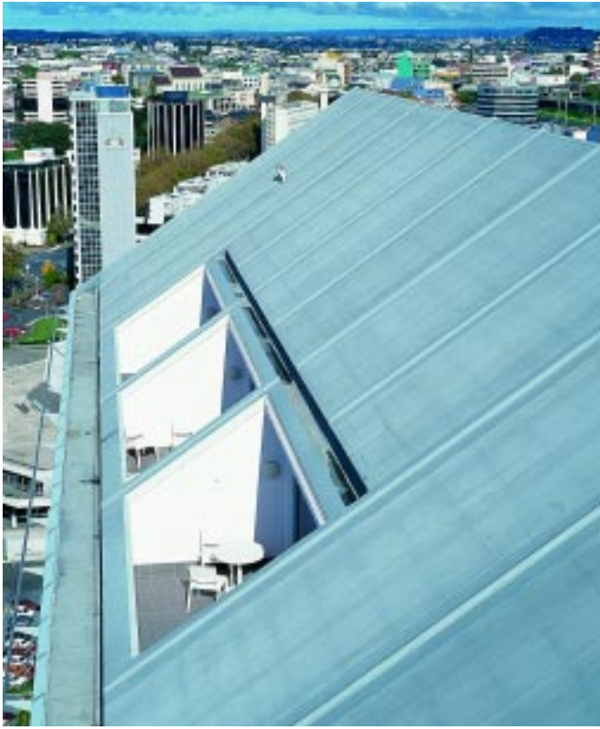
Rubber membrane on plywood
